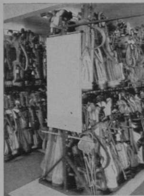
Bag Rack installation in the new pro shop of Ridge CC, Chicago.
