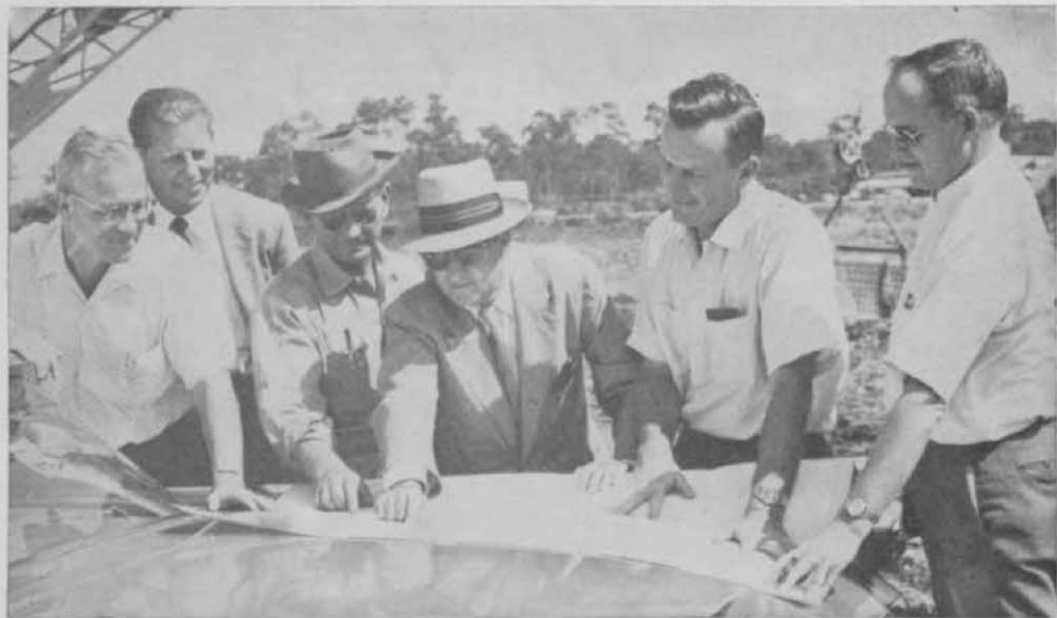
Construction of Palmetto CC, Miami's newest course, was progressing from the blueprint to the building stage when this photo was taken. In it are (l to r): W. M. Porter, one of the owners; Shelley Mayfield, associate architect; O. J. Frank, building supt.; Dick Wilson, architect; and Henry Russell and F. B. Wagor, owners. The course is now being built and will be ready in November, according to present plans. It has two lakes and a 3,000 ft. waterway, giving course 11 water holes. Length ranges from 6,450 to 6,900.
