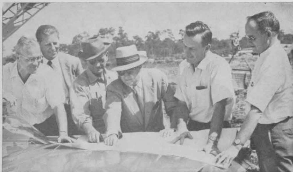
Construction of Palmetto CC, Miami's newest course, was progressing from the blueprint to the building stage when this photo was taken. In it are (l to r): W. M. Porter, one of the owners; Shelley Mayfield, associate architect; O. J. Frank, building supt.; Dick Wilson, architect; and Henry Russell and F. B. Wagor, owners. The course is now being built and will be ready in November, according to present plans. It has two lakes and a 3,000 ft. waterway, giving course 11 water holes. Length ranges from 6,450 to 6,900.
