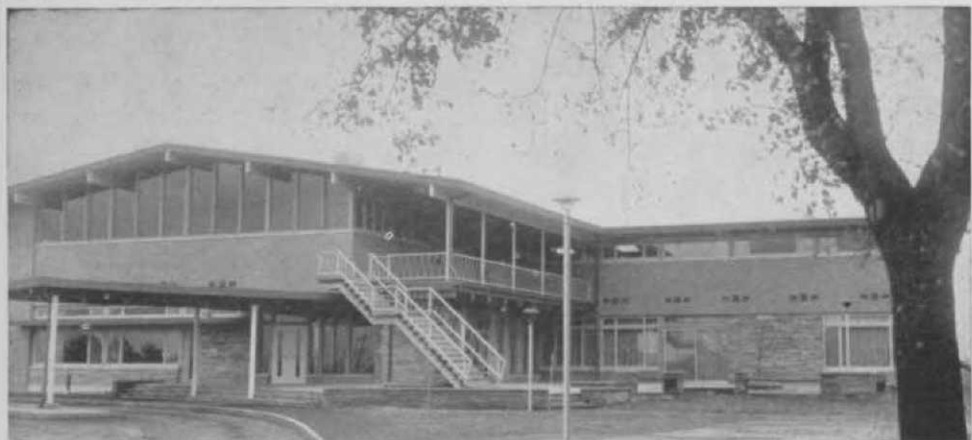
Persons who attend the PGA Championship at Firestone CC, Akron, O., in July will see what is said to be one of the finest clubhouses in the Midwest. It was completed late in 1959 and replaces the building destroyed by fire a year before. Of contemporary architecture, the L-shape building is constructed of Texas brick, Ohio Briar Hill stone and is trimmed in redwood. The first floor is framed by a huge expanse of glass that gives a panoramic view in all directions and the dining room, 40 x 120 ft., extends the entire length of the east side of the building.
