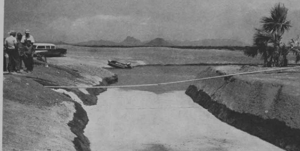
SS-130 is flowed into Indian Bend pond which lost 600,000 gals. of water daily before treatment.
