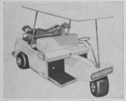
This two passenger Terra-Tire Model #202GT is top car of the new Sloan-Ashland line. Engine is 2cylinder, 4-cycle air cooled Onan; gasoline tank holds four gallans; delivers approx. 18 holes per gal. Wheel base is 751%"; over-all length is 102". The Sloan-Ashland line embraces 10 models, including one, two and four-passenger vehicles, available in either gasoline or electric power. The gasoline cars are offered in one cylinder and two cylinder models, ranging from 4 hp to 12.9 hp.
