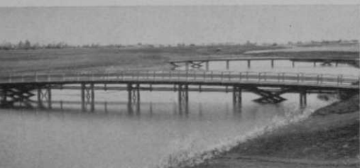
Water is pumped more than 100 ft. uphill to this lake. Two bridges provide convenient access for golfers.
