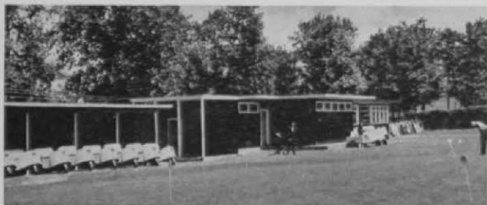
Elmwood CC, White Plains, N.Y. has just completed 20-car garage for club- and member-owned cars. Side windows and roof vents give ventilation. Garage can be easily expanded.
