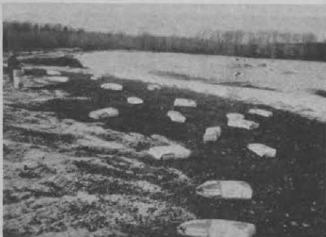
Vermiculite bags are opened and spread over new green areas.
