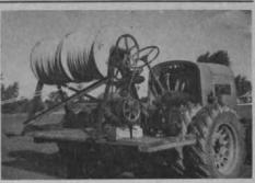
When the Ryder Cup Challenge matches were played at the Wanakah CC, Hamburg, N. Y. last summer it wasn't much of a trick to rope off the fairways and greens. But when the rope had to be retrieved it offered problems until Supt. Al Schardt hit upon the idea of re-winding it with the aid of a winch. It took only six hours to get 45,000 ft. of rope back on the spools.
