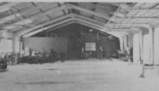
DuBose's workshop and home. 40 by 50 ft. workshop is all rigid steel construction, has bathing facilities for employees, latest in equipment. Home has 3 bedrooms, a den and is located 300 yards from workshop.
