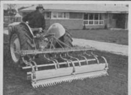
SCARIFIES, GRADES, PULVERIZES, SPREADS, LEVELS, FINISH RAKES
