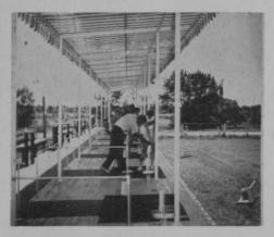
structed like a conventional floor, with joists topped by vertical grain fir flooring sealed with tung oil and painted. The entire base is anchored to a concrete foundation.
