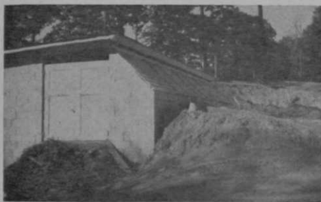
Front of soil processing building, photographed prior to finishing of road areas. The trap doors are for receiving the dumped raw soil.
