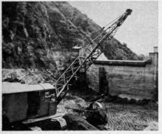
Crane digs soil washed into check dam by floods and loads it into trucks operating on 24-hour schedule. Soil is hauled to Eaton Canyon course and the check dams are cleaned to be in condition for control of future floods.
