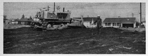
Topsoil hauled from Los Angeles County check dams is distributed over Eaton Canyon course site, saving \$7000 in construction material costs, speeding job and providing interesting undulations. Rocks from the check dam loads are picked out by hand.
