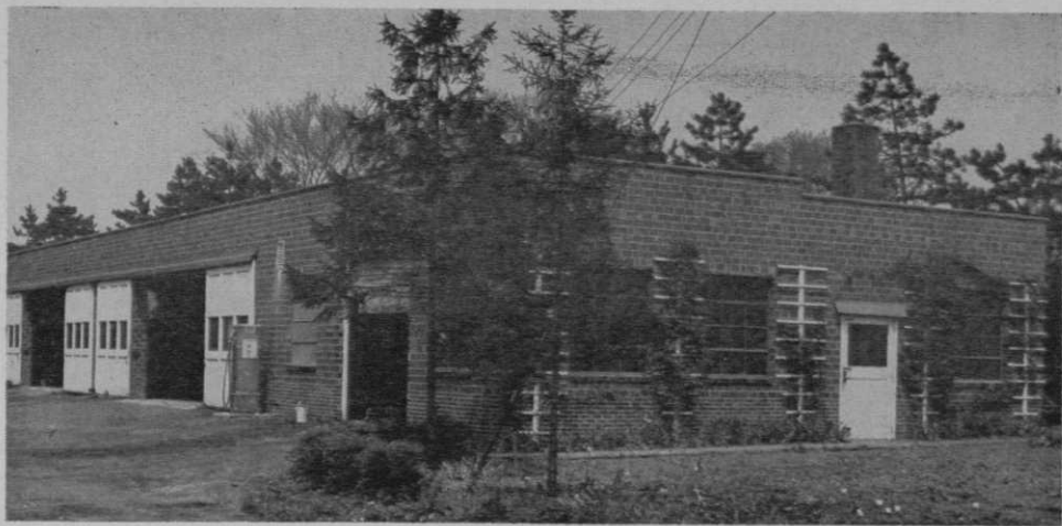
Construction costs were cut by member co-operation in building this new maintenance headquarters at Portage Country Club, Akron, O.
