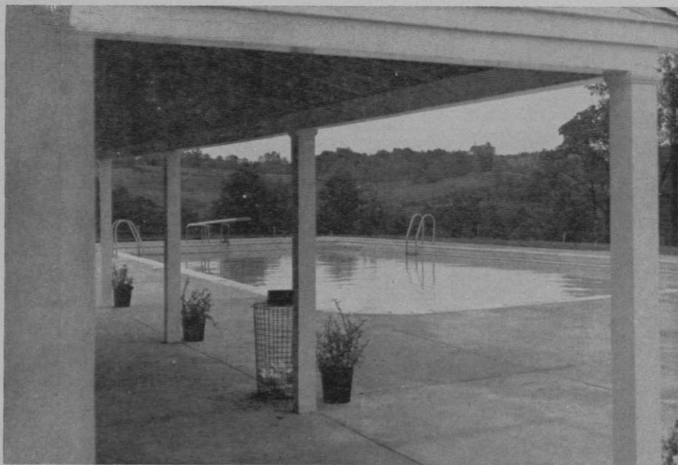
Pool of Indian Valley CC, near Souderton, Pa., is of gunite type construction built by Norris Blue Lake Pool Co. The pool has a beautiful scenic location pleasing swimmers and spectators.
