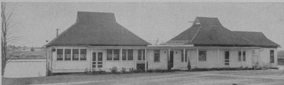
This beautiful little clubhouse between a lake and the first tee, was built from a dirty, dilapidated old structure.
