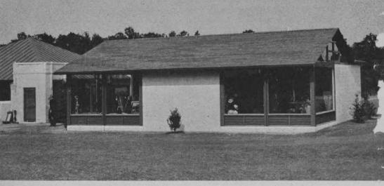
Pinehurst's new pro shop has a lot of window area. Note the ventilators under the windows. These may be opened in summer and closed in cool weather. The four large glass panes under the eaves at the end of the shop are temporary and will be replaced by ventilator fans.
