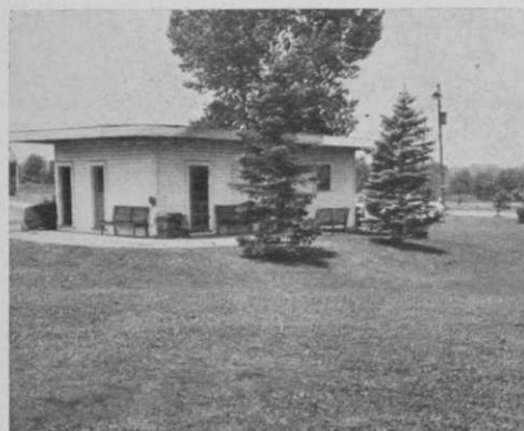
A modest shelter type clubhouse with office, storage and conveniences is adequate.
