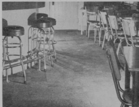
Installation of Do-All corded rubber floor tile.
