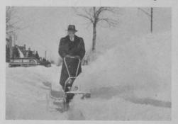
has a 17 in. plowing swath, is powered with a  $2\frac{1}{2}$  Briggs and Stratton 4-cycle engine, is easily pushed and throws snow 10 to 15 ft. to the right or left of the machine. Snow is collected through a screw-action rotor which propels it up and out of the directional shute thus making it impossible for snow to be compacted in front of plow and reducing tendency of the mechanism to freeze in very cold weather.
