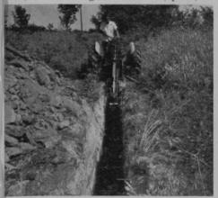
The new Sherman Power Digger is shown cutting an eight-foot deep trench in clay. Rocks and roots made no difference to the digger.
