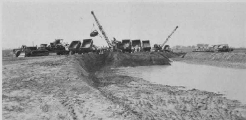
Engineers and operators with earth moving equipment used in excavating lagoon which provided earth for raised greens and serves as a reservoir for water supply which comes from deep wells.
