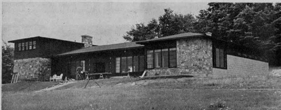
Workmen put finishing touches on Marquette's new clubhouse which faces the first tee and has the ninth green and Lake Superior in the background. Bar is in the corner at the right with men's lockerroom to the rear. Kitchen and women's lockerroom is in left room, below caretaker's apartment on second floor.
