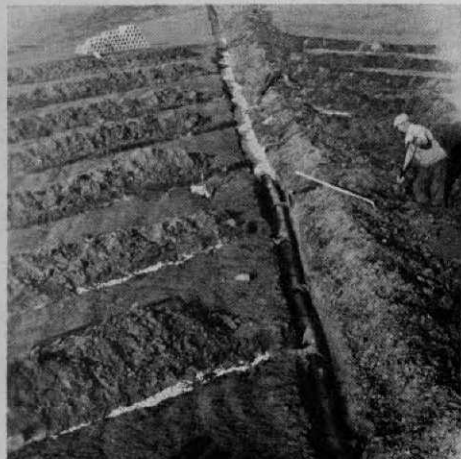
Tiling at 9th hole after line was completed.
