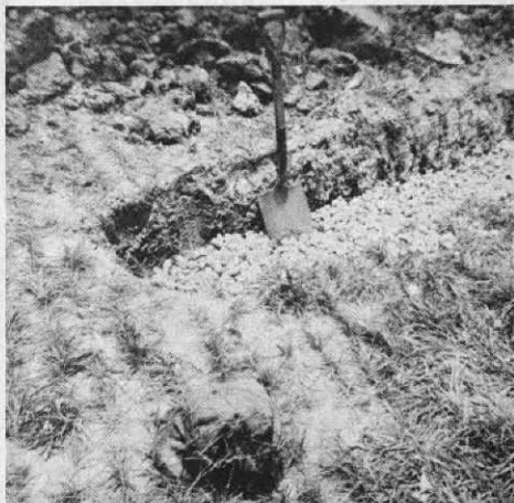
Lateral line after stone backfill; ready for topsoil.
