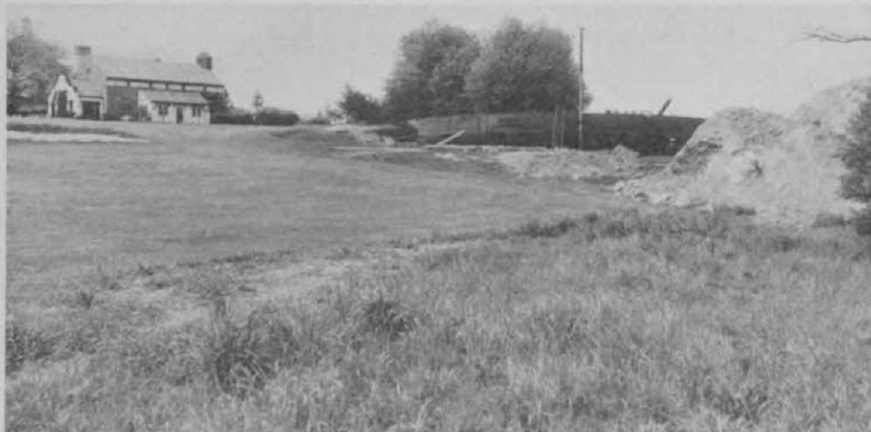
The giant 300,000-gallon tank installed by Bethlehem Steel at the North Hills Golf Club, Long Island, within New York City, is seen above back of the eighteenth green, with the Moorish clubhouse in the left rear. It required more than two months of constant digging before the plumbers, electricians and welders moved in to complete the $25,000 operation. The New York City courses have been denied the use of water except for their clubhouses.
