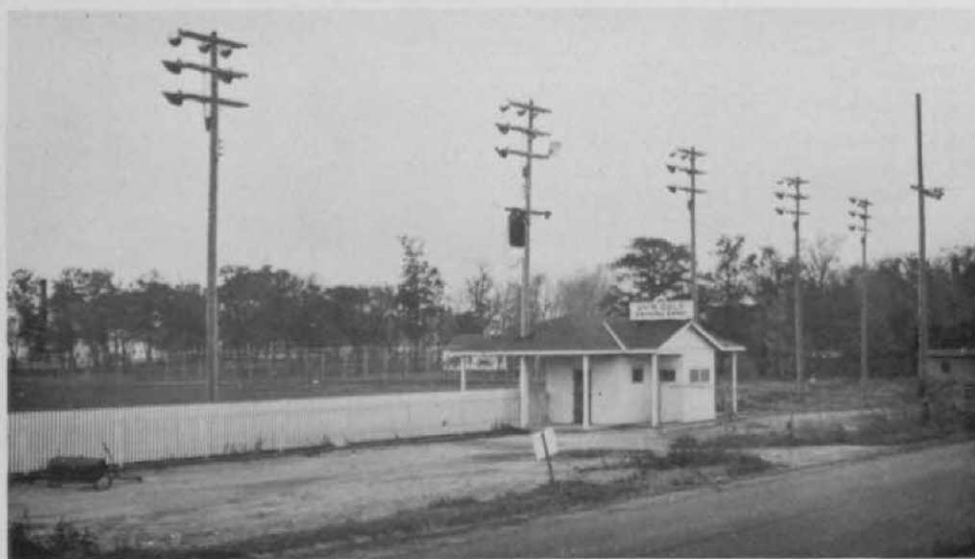
The small clubhouse at the Univ. of Minnesota Driving Range has been designed to control all player traffic to and from the tees and original plans have been altered to provide parking space directly back of the tee line for spectators and guests who accompany players.
