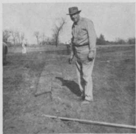
Heavy work of installing watering system was complete when ditch was filled and packed and turf relaid.
