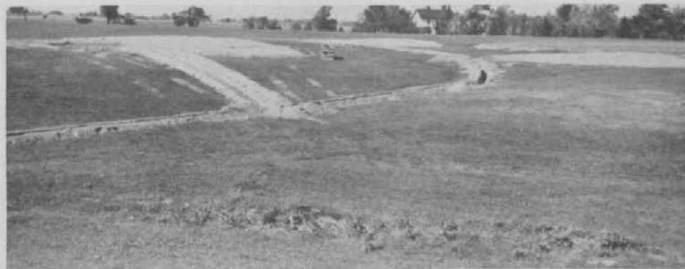
Drainage of traps around this new green (right rear) is being taken care of by tying them into the main tile system.
