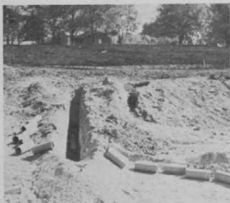
Tile was laid in the sub soil of this new green before the top soil in background was applied.
