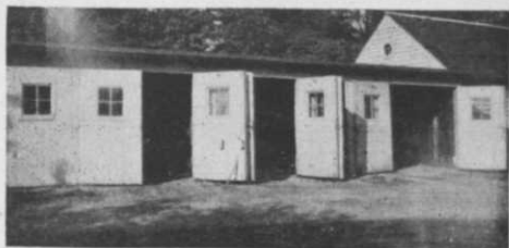
Maintenance garage at Canterbury.
