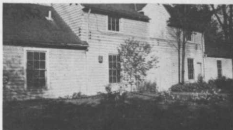
Storage space, shop and facilities for supt. and staff are located in Canterbury's maintenance building.
