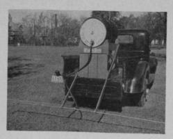
50-gallon gravity feed spray unit that can be built quickly, easily and economically in the shop of any greenkeeper from materials usually on hand.
