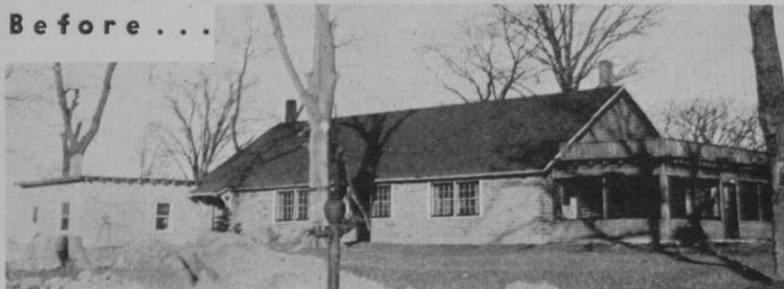
View of the old Marion clubhouse before its transformation.
