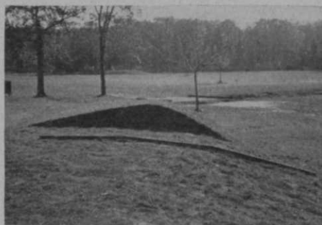
Fig. 2—Regraded bank in foreground is shown by gauge to be right for machine mowing. Compare with original grade at rear.
