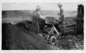
It's thumbs down on raking, screening and picking out trash by hand at the Hieland Golf Club, Watseka, Ill. Their Model "K" Royer shreds sod, compost, sludge and other materials, reducing it to pea size particles that readily spread and quickly yield nutrients to bent and grass roots.
