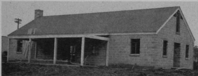
Photo of Tam O'Shanter caddie house, taken shortly before completion of the structure. The completed building is finished in white, with green roof, to match the main clubhouse.
