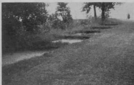
To defeat side-hill wash, these stepped-down sand traps skirt the fairway edge on one of the Klinger Lake holes. Previous to their construction, Millar had great trouble maintaining turf in this area.
