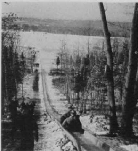
Toboggan slide at Passaic County (N.J.) GCse, where Kent Bradley superintends, is extremely popular with winter sports enthusiasts in the vicinity. Slide, which was built by WPA workers, is 300 ft. long; tobogganers enjoy another 700-900 ft. slide on the fairway after leaving the incline.
