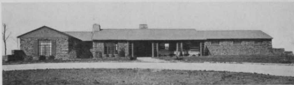
Amarillo's new clubhouse for many course golfers, which has just been completed, provides ample shower and locker facilities, plus plenty of lounging space; cost was $17,500.
