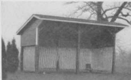
Shown above is the new practice driving shed constructed this year at the Whitmarsh Valley CC in the Philadelphia District. The cost of the shed was around $300, according to Pro Morrie Talman. Morrie is now able to give lessons at any time, rain or shine, and can also provide an added bit of privacy for students taking lessons from him. The practice shed has been 'well worth the cost,' Morrie says.
