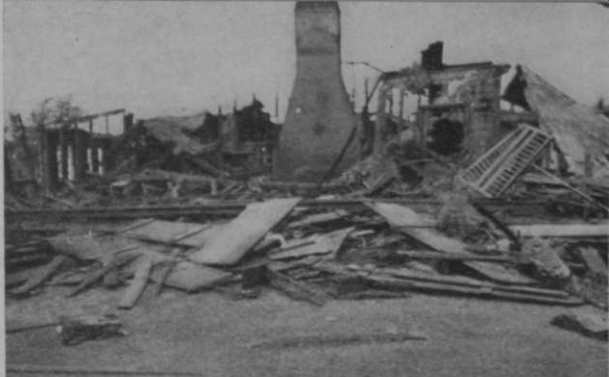
What was left of the clubhouse at Bear Hill GC, Stoneham, Mass., where Leslie Cottrell is pro-mgr., after a fire on Sept. 8.
