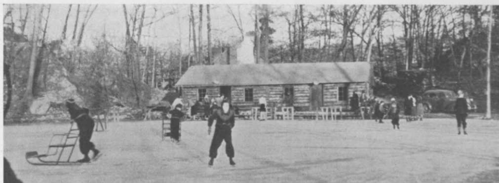
At the Charles River CC, Newton Centre, Mass., this rink attracts large winter patronage. Cabin is warming house for shelter and dressing.
