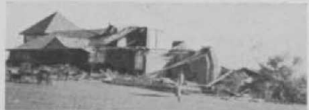
At Leicester, Mass., the hurricane demolished half the clubhouse.
