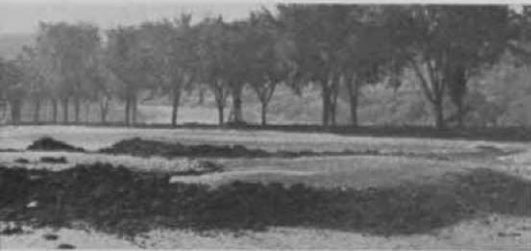
Two to ten inches of river silt being removed from green and fairway at Tekoa CC, Westfield, Mass.
