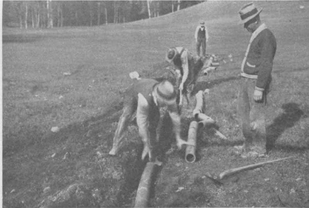
A short shallow tile line through a low wet portion of fairway costs little and helps the turf as well as playing conditions in wet seasons.
