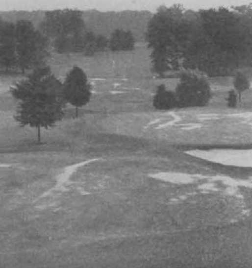
Poor surface drainage is indicated by the puddles of water on important turfed areas of this course.
