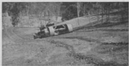
Tractors proved indispensable in grading and shaping both fairways and greens.
