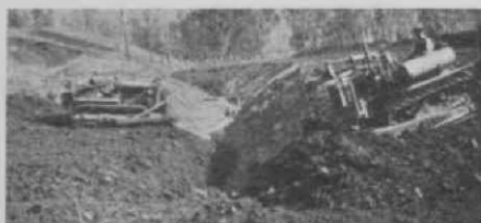
Tractors are seen here filling ditch before 13th and 18th greens.
