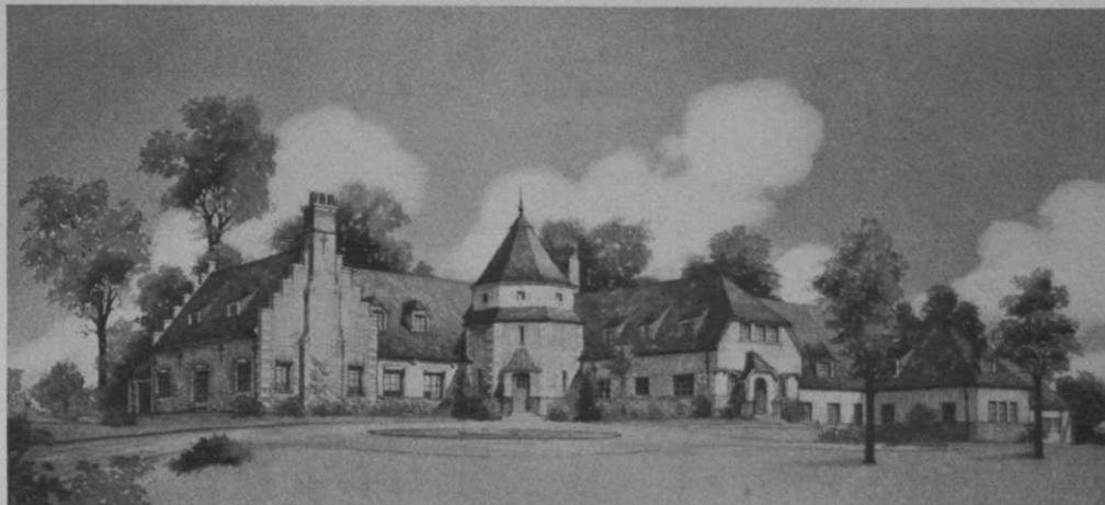
New clubhouse of Cascade Hills CC, Grand Rapids, to be formally opened early in the summer, replaces clubhouse destroyed by fire. Clifford C. Wendehack, specialist in country clubhouses, is architect. Among distinctive features are a Nineteenth Hole in connection with men's locker-room, and far more space for women than generally is found in older clubhouses. The Nineteenth Hole has a high ceiling of acoustical materials to absorb the din of the whoopee and the moan of the "shoulda had's."
