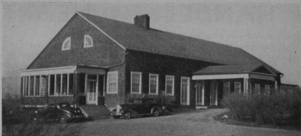
Although not as beautiful as some club structures, Carlisle's members are proud of their clubhouse, built from two large barns, which measure 50 x 110 ft. Building has three large porches, with locker-room and 'Pine Room' located in basement.
