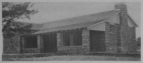
Above is the recently completed clubhouse of the Tishomingo (Okla.) CC. This building is of native stone, the labor being done by local men under supervision of the WPA. The building consists of a main room 24' x 30', two locker rooms and kitchenette. A stone fireplace is located in the main room.
