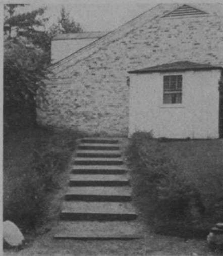
These steps leading to Orchard Lake's locker-room are dense as concrete, but are made of 'stabilized' soil.
